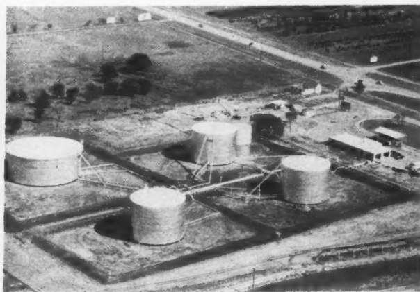
IRVING TERMINAL, located between Dallas and Fort Worth, is the end of the line, serving the North and West Central areas of Texas.
